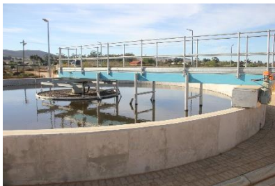
Secondary Settling Tanks
