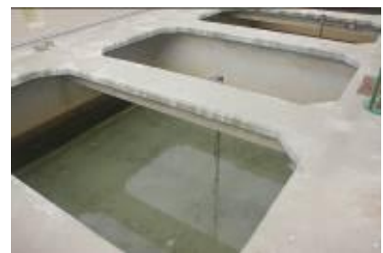
Rapid Gravity Sand Filters
