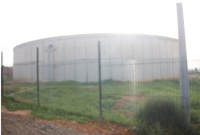
4.000 MI Wesbank Reservoir No. 4
