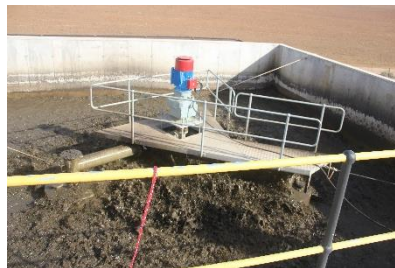
Aerobic Digester with floating aerator
