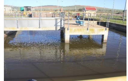
Bio Reactor: Anoxic zone
