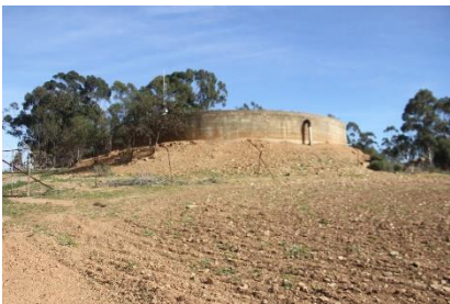
2.554 MI Moorreesburg Reservoir No. 3
