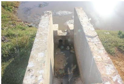
Inlet at Primary Pond
