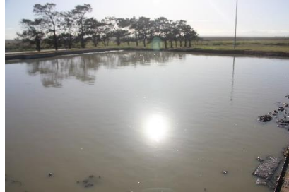
Anaerobic Pond No. 1
