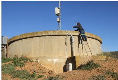
0.275 MI Koringberg Reservoir No. 2
