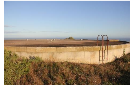
2.553 MI Yzerfontein New Reservoir
