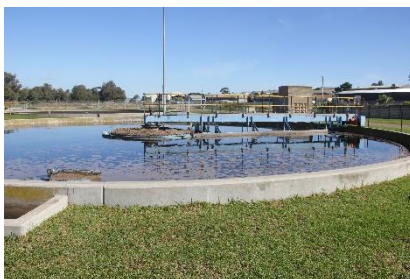
Secondary Settling Tank No. 1
