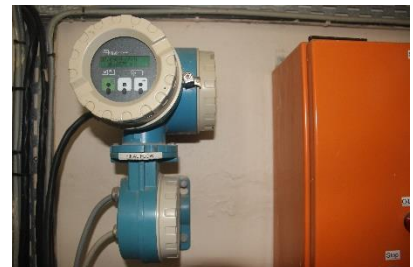
Kasteelberg Reservoirs at Swartland WTW
