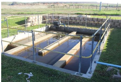
Chlorine Contact Channel
